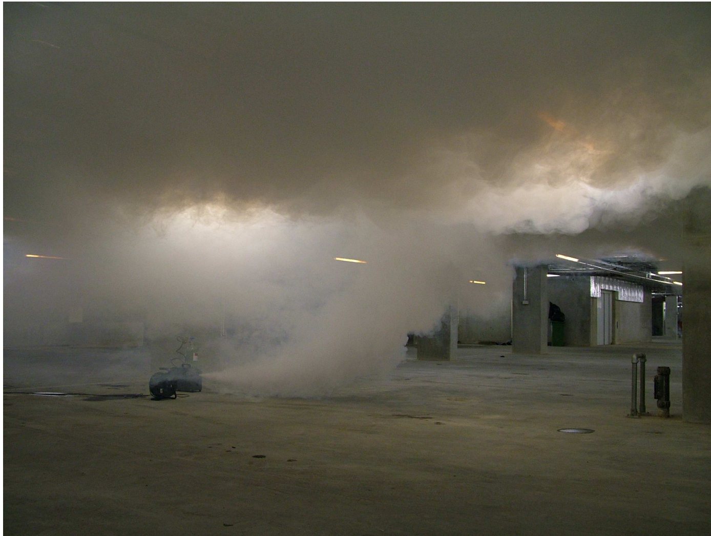
Emergency Ventilation – Smoke Test
